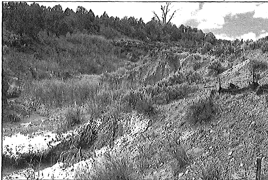
Figure 2: Looking upstream of leak site and hillside to the east where the site will be accessed.
